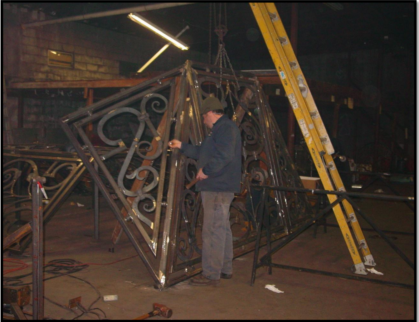
Here the canopy is being disassembled. The welds are being inspected for quality and finish by owner blacksmith Timothy Miller.
