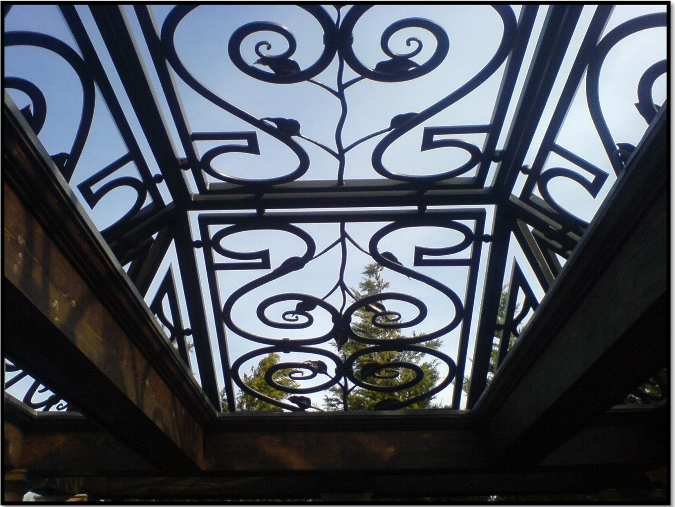
Here is view from the inside.
