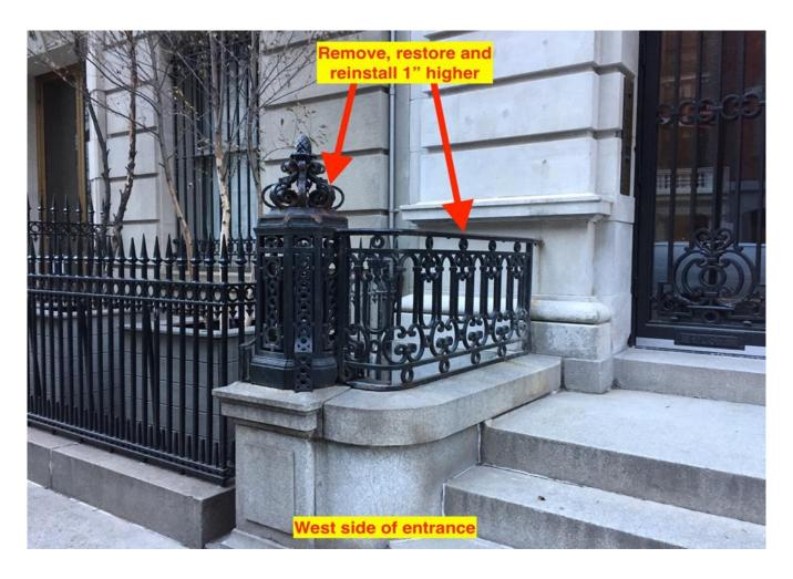
Here, you can see the original scope of work that was needed to restore the original ironwork. The plans were provided to us by the G.C. and required by the client and the New York City Landmarks Preservation Commission.
