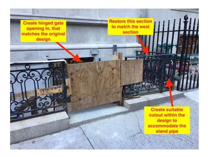
This project was multi-faceted. It involved recreating, restoring, and refinishing various parts of the ironwork. This included the exterior railings, gates, handrails, and decorative newel posts. Our first process was to carefully inspect and inventory all the parts that were to be removed and brought back to our studio for restoration.
