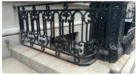
These images illustrate a portion of the corrosion and damage found throughout the ironwork. We also discovered marks of an earlier restoration which was poorly executed. We would have to redo the previous work to restore the ironwork to its previous glory.
