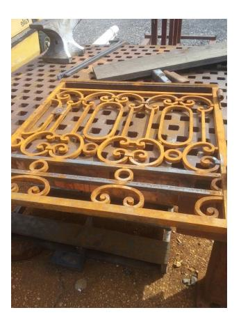
Here are a few images showing the ironwork in various states of repair. The top image shows pieces of additional cap moulding which were custom bent to fit the top of the railings. The gate section (seen on bottom left), was in bad shape. In addition to repairing its existing damaged areas, we re-made areas that were missing and/or too damaged for restoration. Finally, we replaced the original hinges and steel gate latch with custom ones made at our studio.
